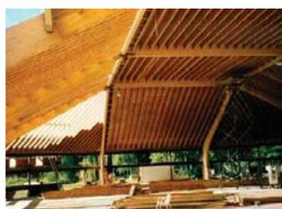
Birchwood Community Church in Anchorage, Alaska. These glulam arches were sized to achieve a one-hour rating. The roof-ceiling assembly will have two layers of 3/4-in. (16mm) gypsum wallboard attached to the bottom of the roof joists. The steel connections will be covered with 2x wood blocking.
