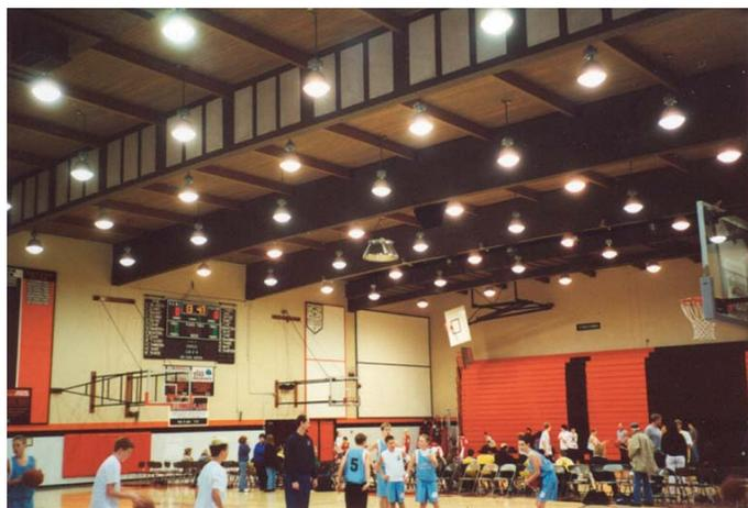
High school gymnasium with heavy timber roof. Notice the large main and secondary beams and 2 x 6 (38 x 140 mm) tongue and groove decking.
