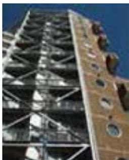
uncommon in Canada, such systems may provide an excellent model for tall timber hybrid buildings. The 12-story Scotia Place in New Zealand is a good example of a timber-steel hybrid.
