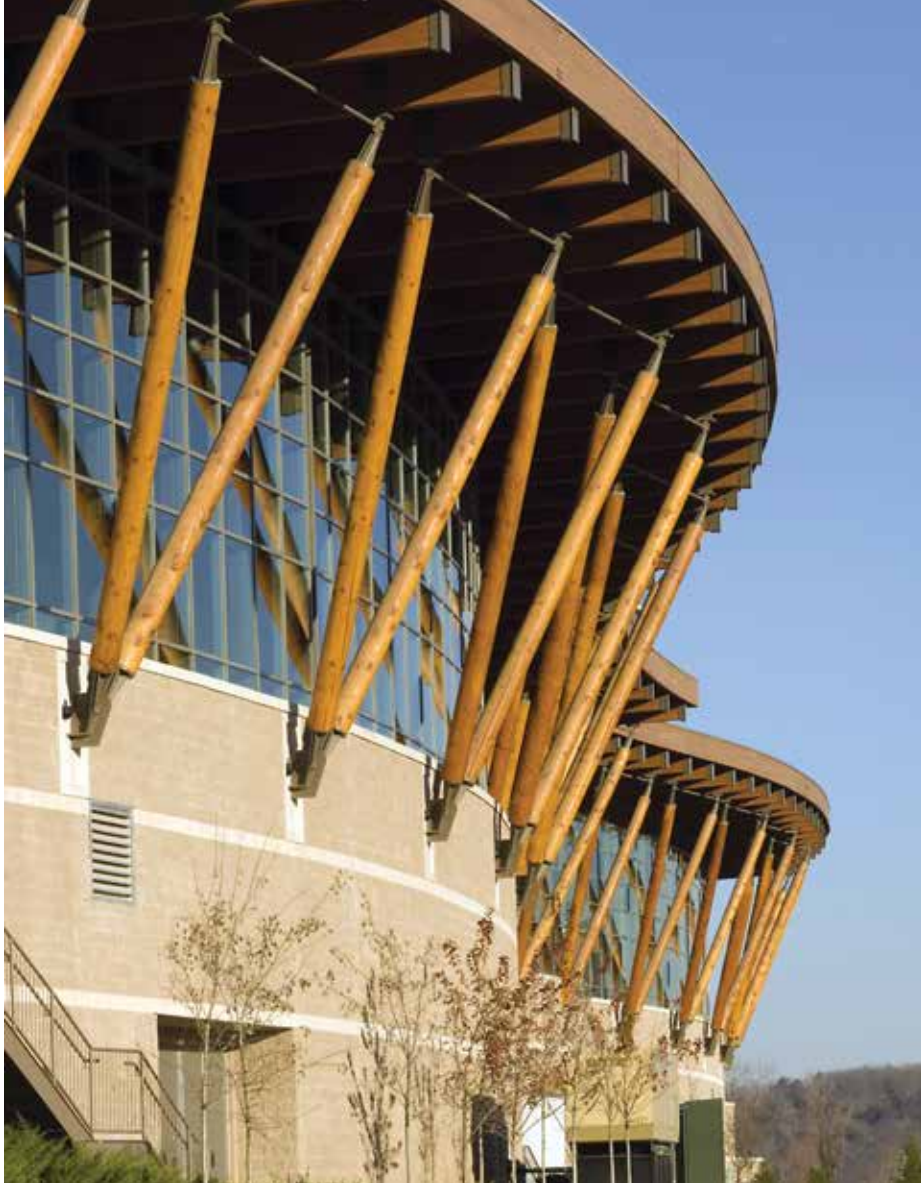
Designed by tvsdesign, the Branson Convention Center in Branson, Missouri, features a large overhanging roof. By sheltering the wood underneath, the roof deflects precipitation and helps to ensure long-term durability.
