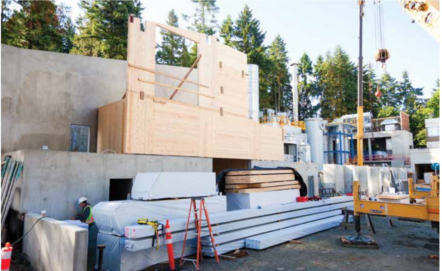
Once delivered to the construction site, wood should be stored and wrapped properly.
