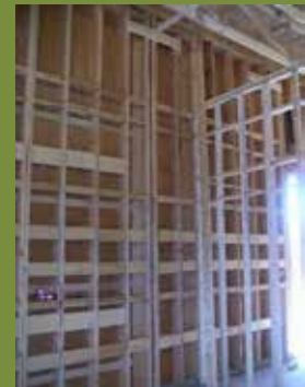
This jewelry store in Tennessee includes 22-foot walls made from 2-by-8 Douglas-fir. Prefabricated off-site, the walls were delivered with insulation and brick veneer already installed.
