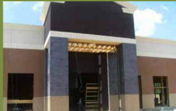
This jewelry store in Tennessee includes 22-foot walls made from 2-by-8 Douglas-fir. Prefabricated off-site, the walls were delivered with insulation and brick veneer already installed.
