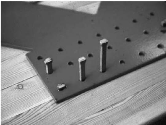
Figure 1.—Typical timber rivet connection.
