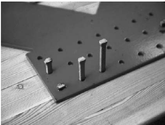
Figure 1.—Typical timber rivet connection.
