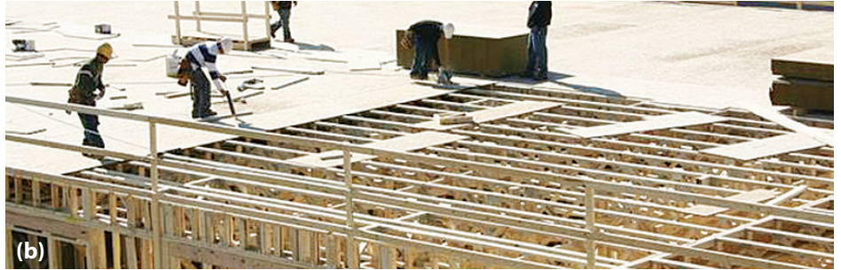
Figures 3a and 3b. Periodic special inspection is required for nailing, bolting, anchoring and other fastening of elements of the seismic and main wind force-resisting systems, including wood shear walls, wood diaphragms, drag struts, braces and hold-downs.
