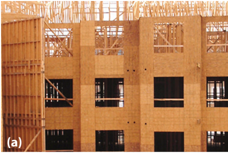
Figures 3a and 3b. Periodic special inspection is required for nailing, bolting, anchoring and other fastening of elements of the seismic and main wind force-resisting systems, including wood shear walls, wood diaphragms, drag struts, braces and hold-downs.
