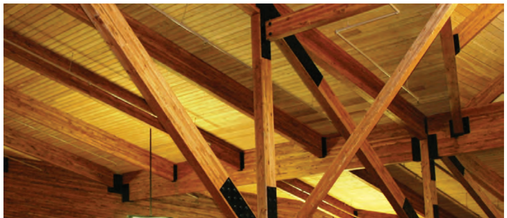
Glulam beams used in roof system.
