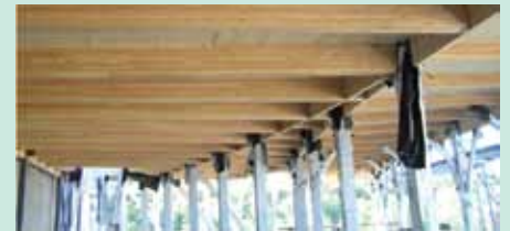
The Promega biotechnology production facility features an innovative mix of glulam and cross laminated timber.
