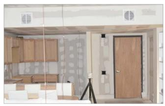
Figure 28. HVAC duct openings in drop ceiling.
