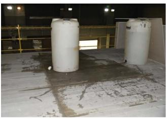
Figure 55. Water tank that leaked.
