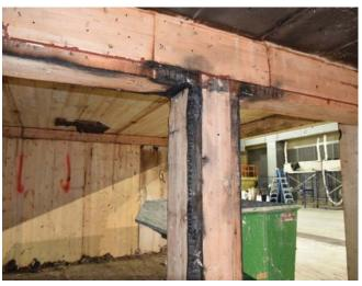
Figure 65. Damage to support column and midspan beam.
