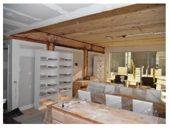
Figure 36. Exposed cross-laminated timber ceiling and glulam support columns and beams in the living room for Tests 4 and 5.
