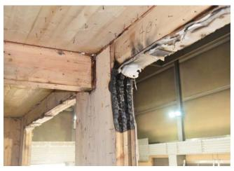
Figure 61. Localized section loss caused by charring on Wall A at the living room opening on the second floor.
