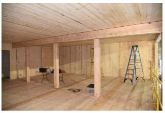
Figure 19. Support beam and columns on the second floor.
