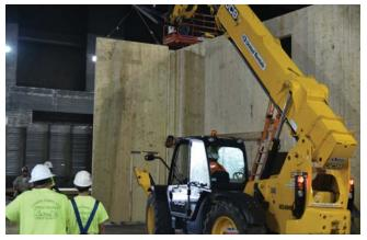
Figure 4. Installation of a cross-laminated timber wall panel.
