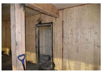
Figure 63. Localized section loss caused by charring around apartment door frame on the second floor.
