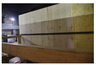
Figure 7. Steel angle located on Wall B to support the second-level floor in the apartment.
