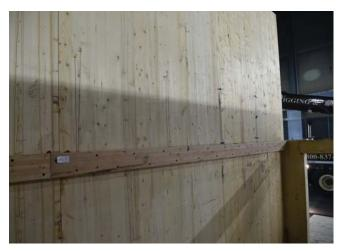
Figure 10. Ledger on Wall D to support second-level floor in the apartment.
