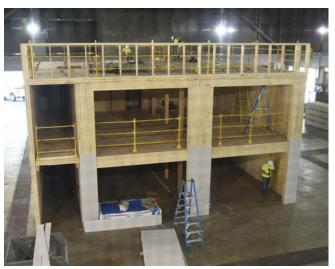
Figure 20. Partial wall constructed along the top of Wall A.
