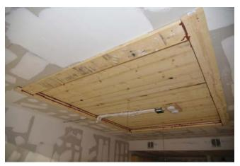
Figure 33. Exposed cross-laminated timber ceiling in the living room for Test 2.
