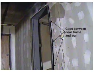
Figure 99. Gaps between door frame and wall.
