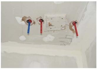
Figure 32. Plumbing penetrations in the utility room on the first-floor level.
