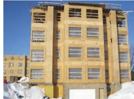
Figure 3: Type V Construction
