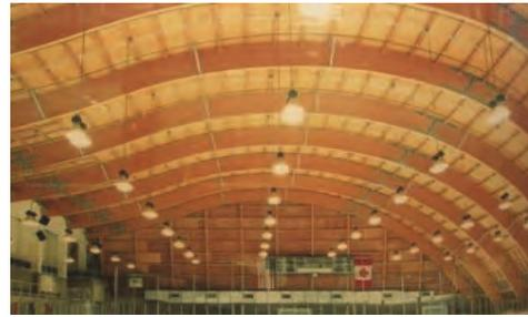
Figure 13: Heavy Timber Construction
