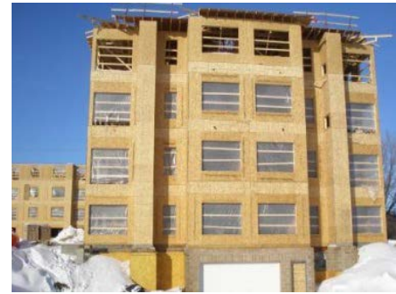
Figure 2: Type V Construction
