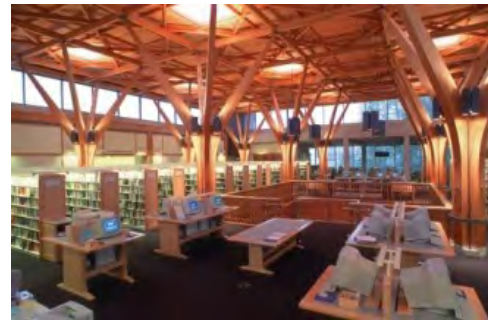
Figure 3: Type IV Construction
