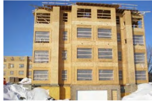
Figure 2: Type V Construction
