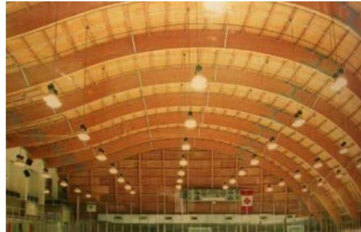
Figure 13: Heavy Timber Construction
