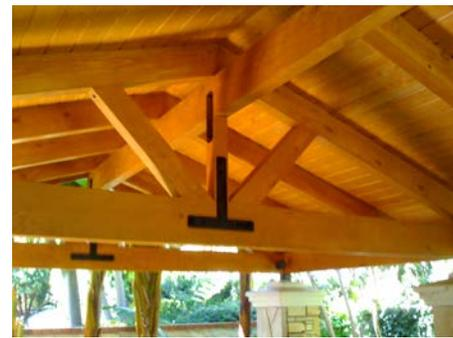
Figure 3: Type IV Construction
