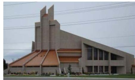
Figure 4: Type III Construction
