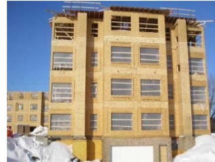
Figure 2: Type V Construction
