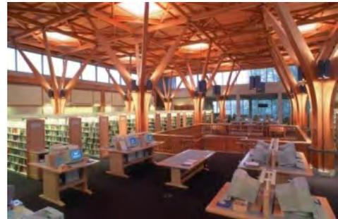
Figure 3: Type IV Construction
