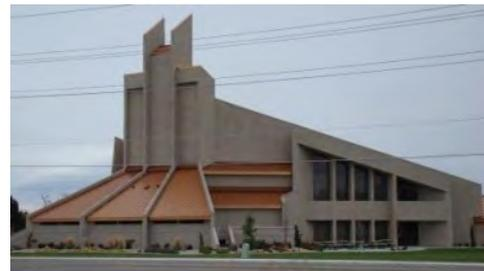
Figure 4: Type III Construction
