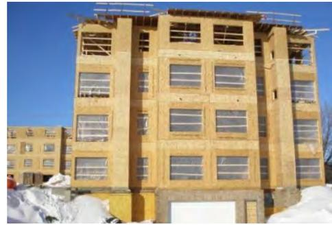
Figure 2: Type V Construction
