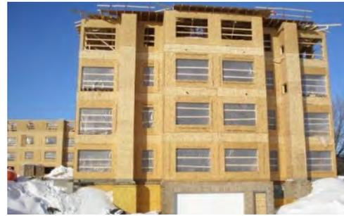
Figure 2: Type V Construction
