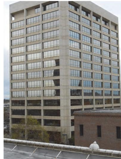
Figure 5: Type I Construction
