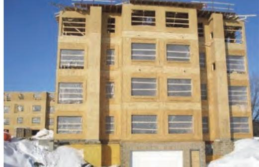
Figure 2: Type V Construction
