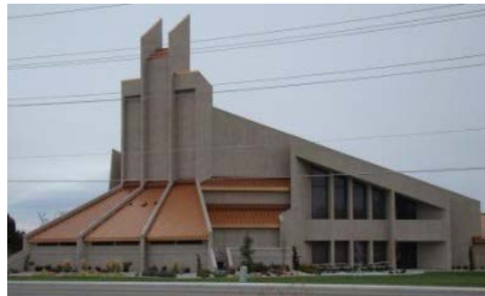
Figure 4: Type III Construction
