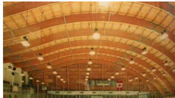
Figure 12: Heavy Timber Construction
