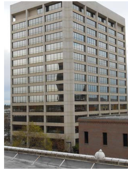
Figure 5: Type I Construction
