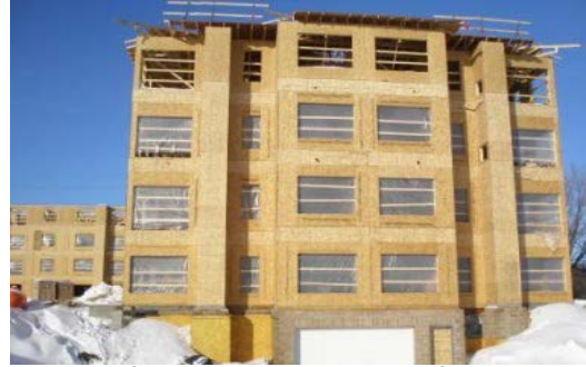
Figure 2: Type V Construction
