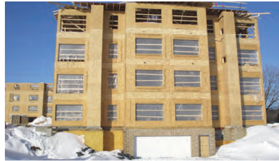
Figure 2: Type V Construction
