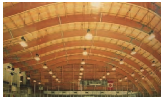
Figure 13: Heavy Timber Construction
