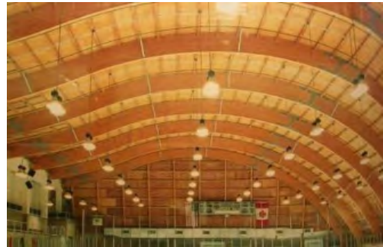
Figure 10: Heavy Timber Construction
