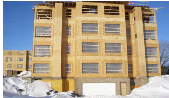
Figure 2: Type V Construction
