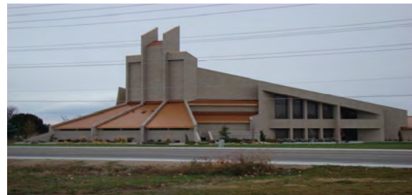
Figure 4: Type III Construction
