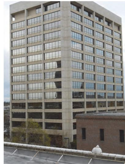
Figure 5: Type I Construction
