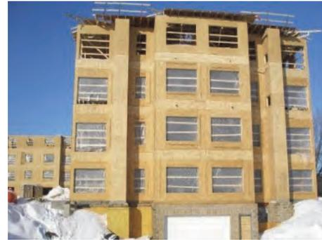
Figure 2: Type V Construction
