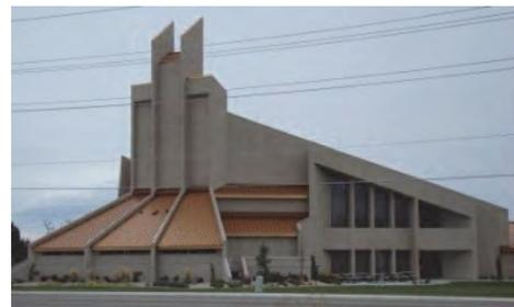
Figure 4: Type III Construction
