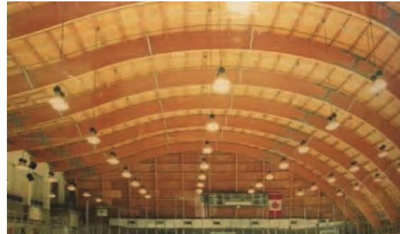
Figure 13: Heavy Timber Construction
