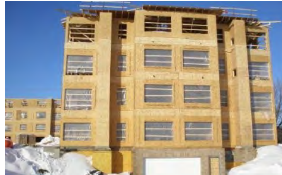
Figure 2: Type V Construction
