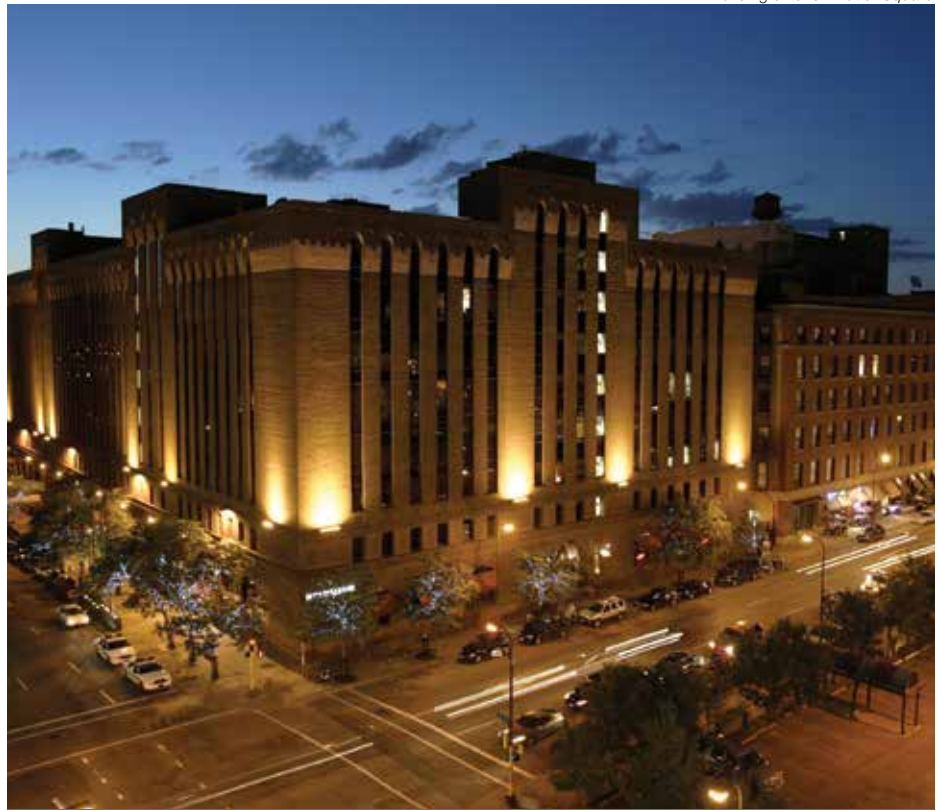
Building exterior: Butler Square
