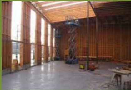
This restaurant in California includes 24-foot walls made from 2-by-8 Douglas-fir.
