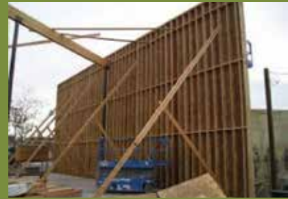
This restaurant in California includes 24-foot walls made from 2-by-8 Douglas-fir.
