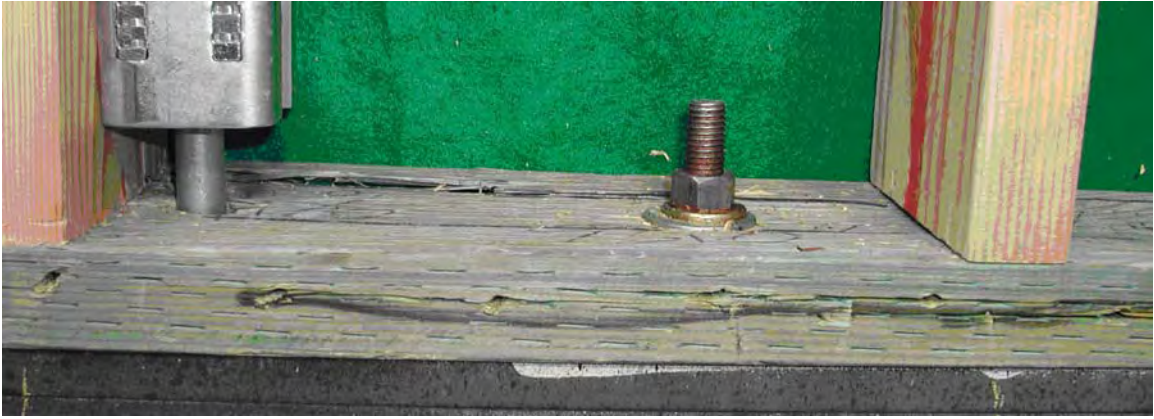
Figure 13. Splitting along narrow face on west side of wall (Wall G2)
