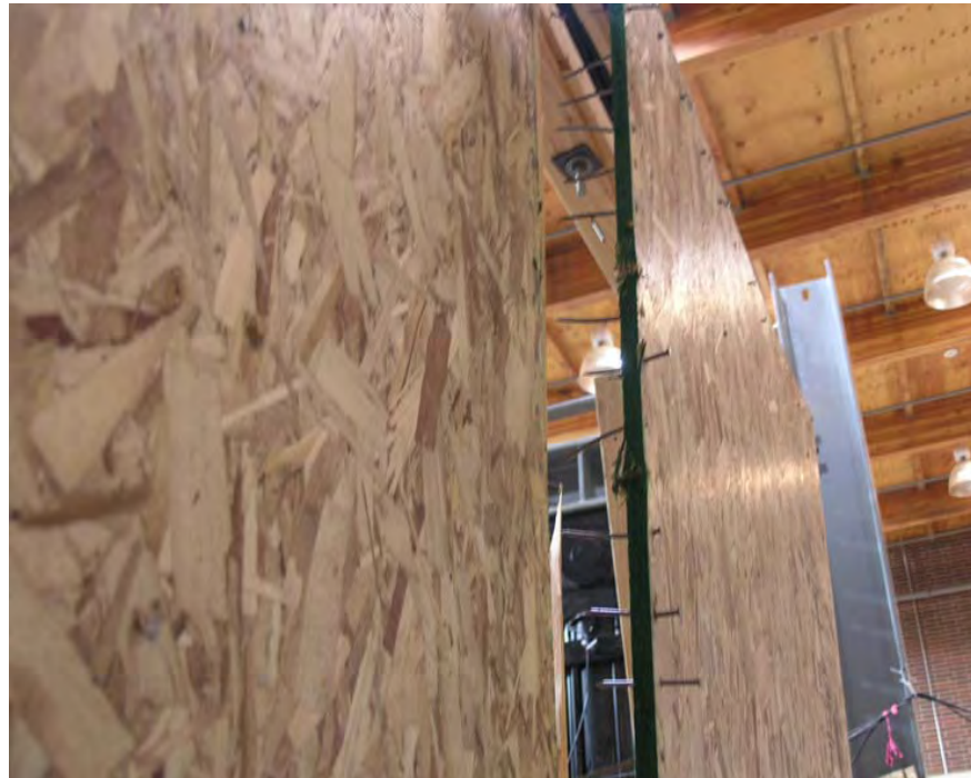
Figure 18. Slight yielding of nails around the perimeter (Wall H1)
